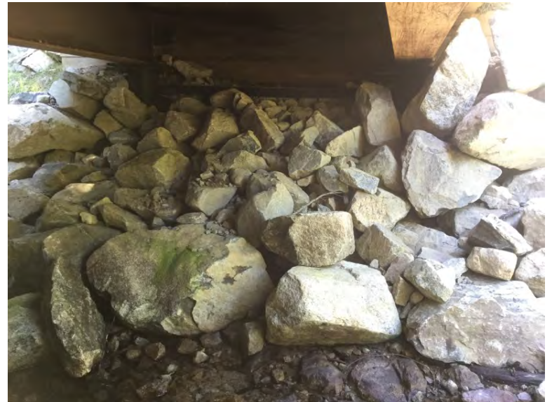
Right Bank Abutment when facing downstream
