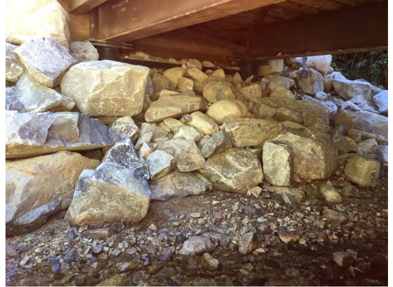
Left Bank Abutment when facing downstream
